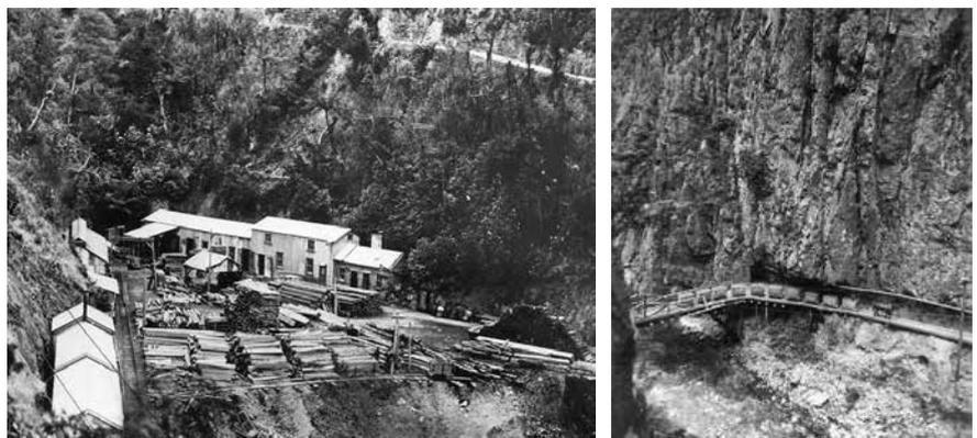
Mining operations were conducted over 10 levels with the lowest level, 5B, being some 100m below the level of the Waitawheta River.
